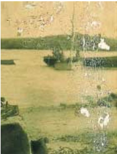
The emulsion is badly cracked and is beginning to peel away from the paper base.
